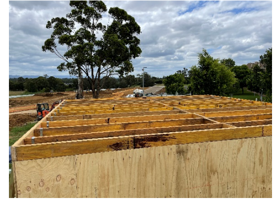
Framing for viewing platform
