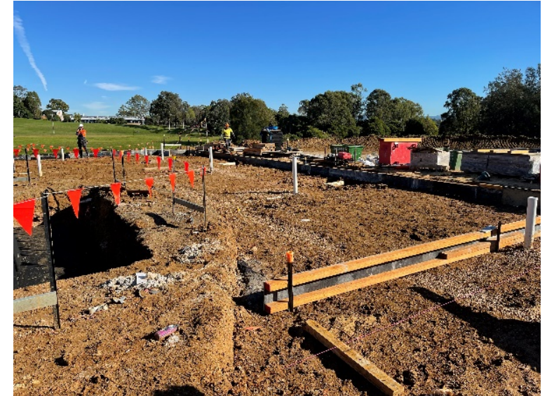
Lower ground floor form work edge boards
