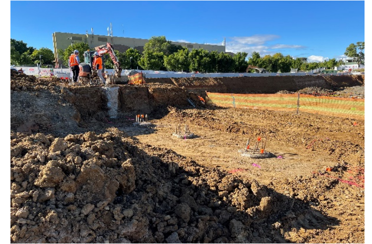
Detailed excavation of capping beam to Northern shoring wall
