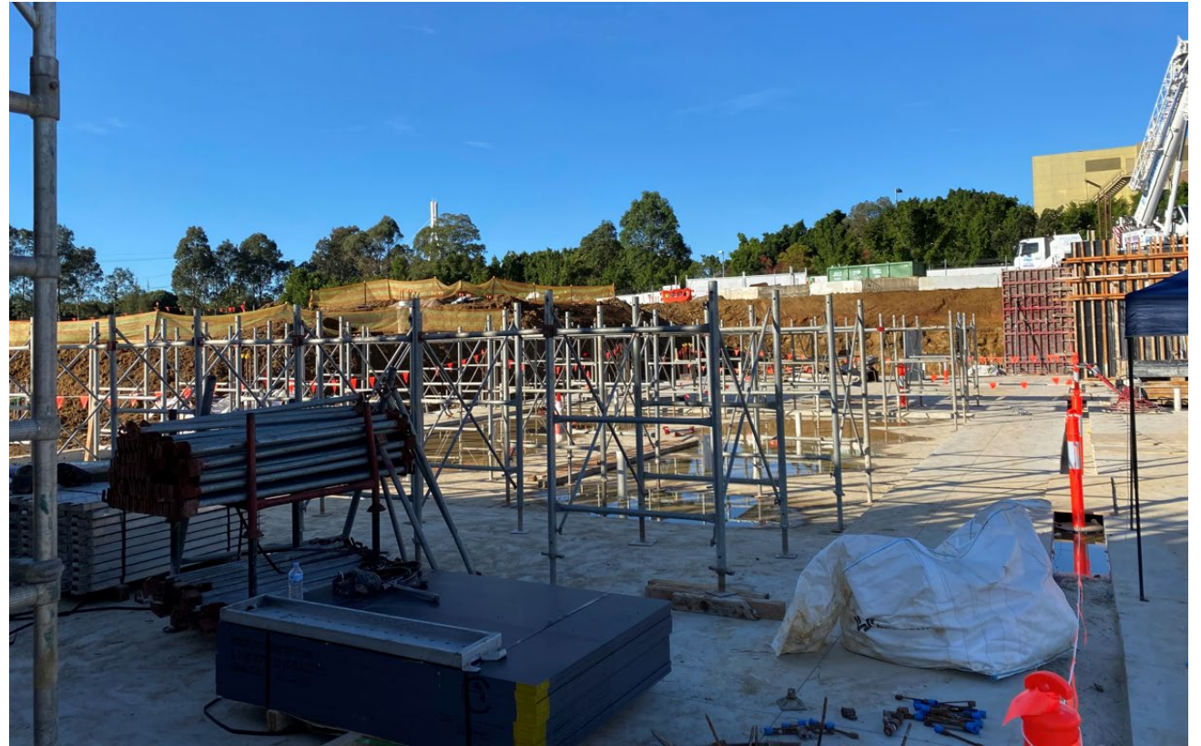
Upper ground floor frames for deck being placed
