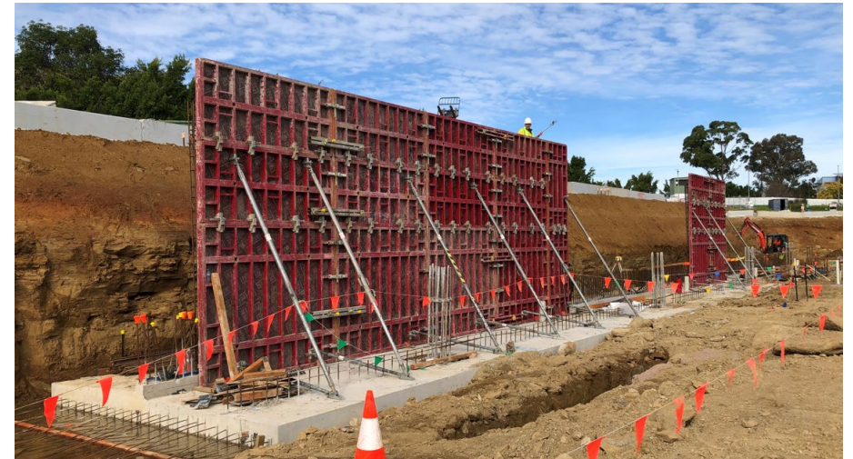
Retaining wall shutters
