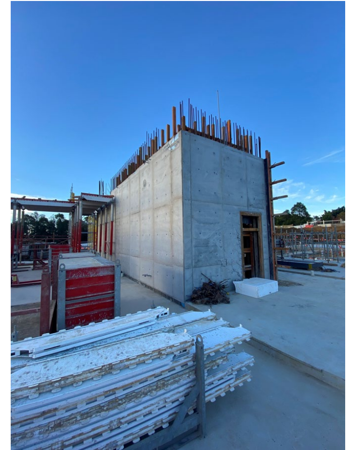
Stair core 01 stripping underway and high strutted formwork commenced
