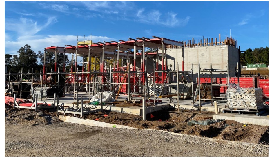
Stair core 01 and high struted formwork
