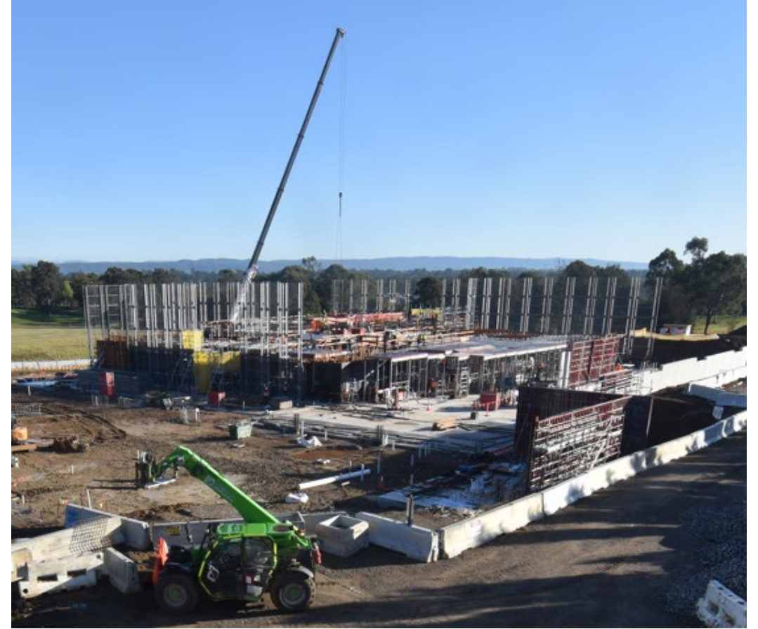
Erection of formwork perimeter safety screens
