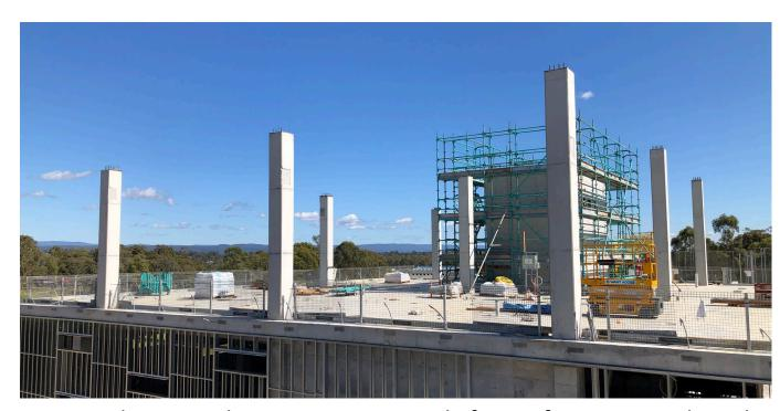
L1 columns and stair core No.1 ready for roofing structural steel
