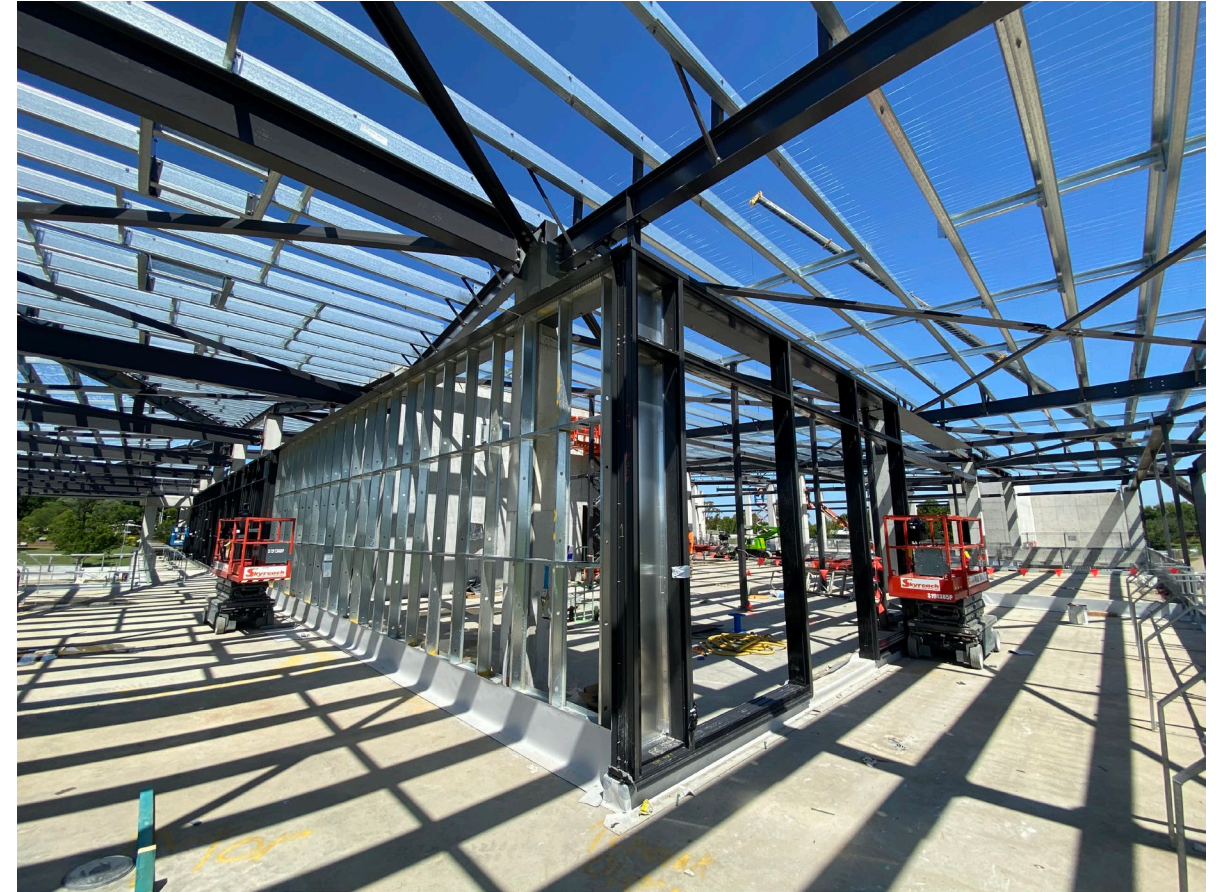
Level 1 Glazing and façade framing
