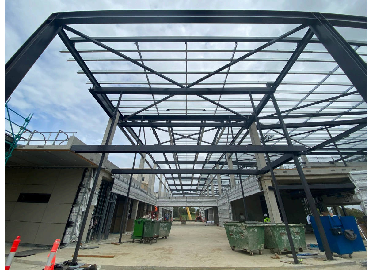
Central Atrium roofing steel
