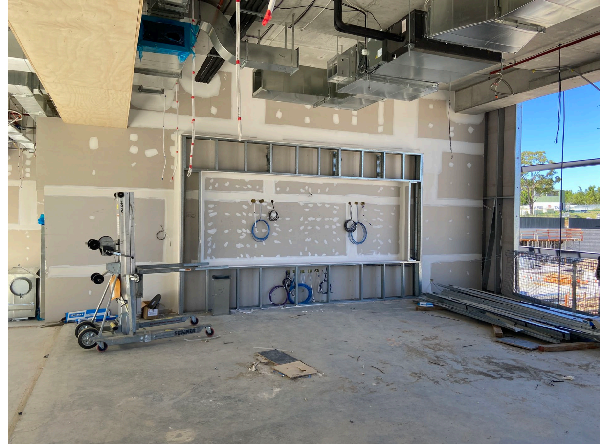
Internal wall framing and sheeting
