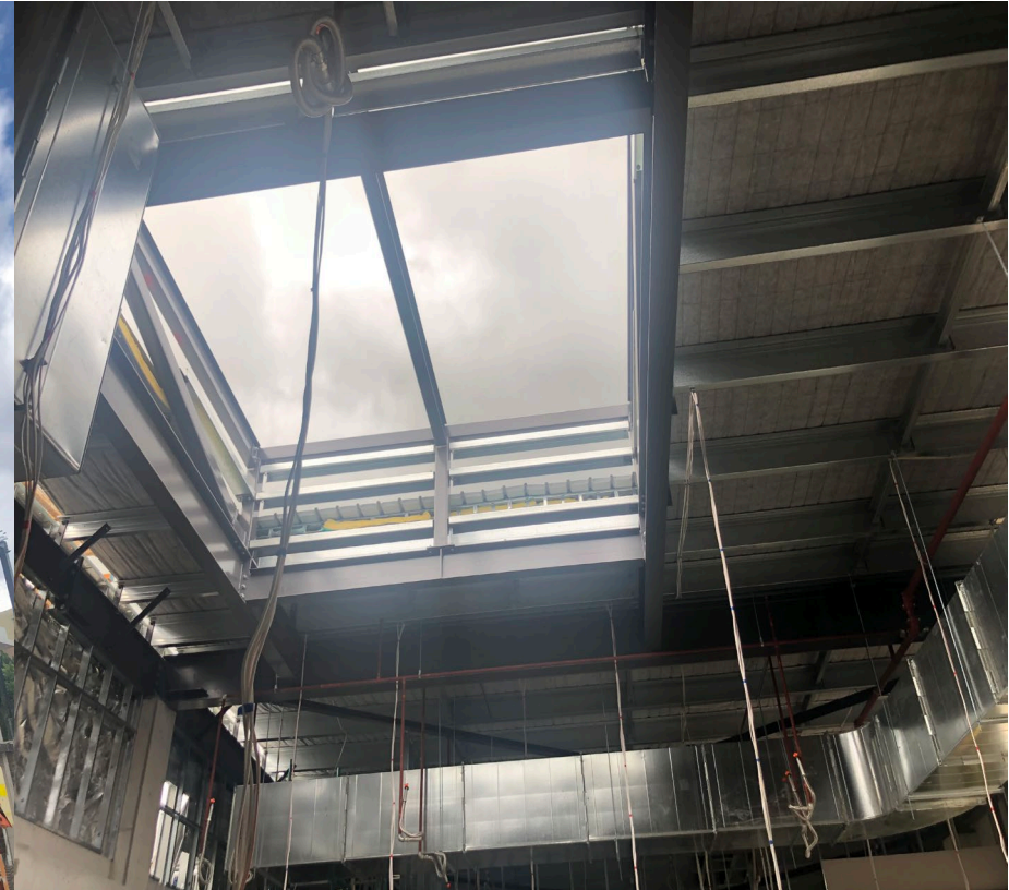
Northern Skylight Opening and High-level Service Rough-in
