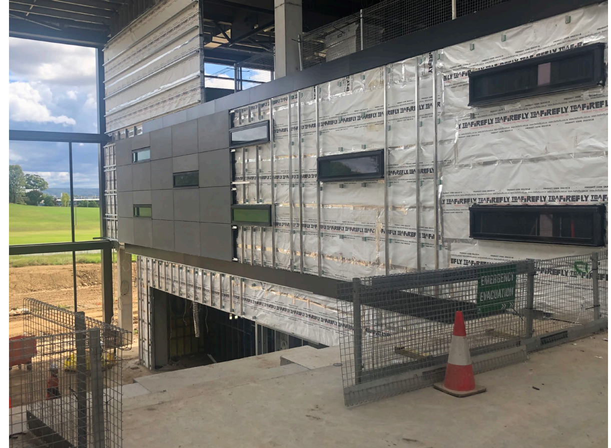
Central Atrium Internal Panel Installation
