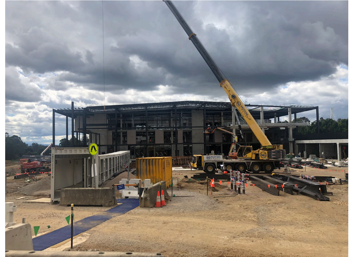
Northern Aspect Structural Steel Installation
