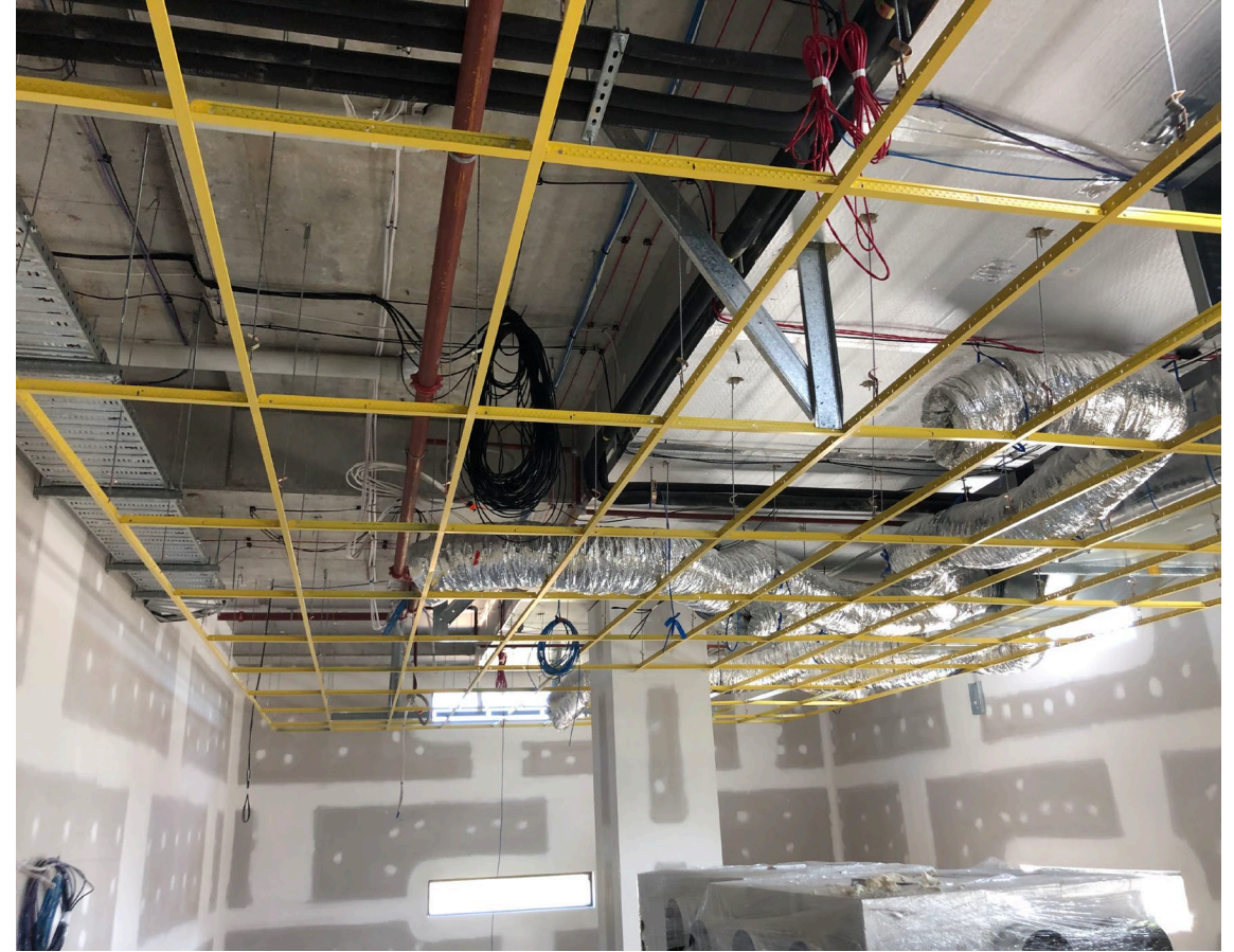
Internal Ceiling Grid Installation
