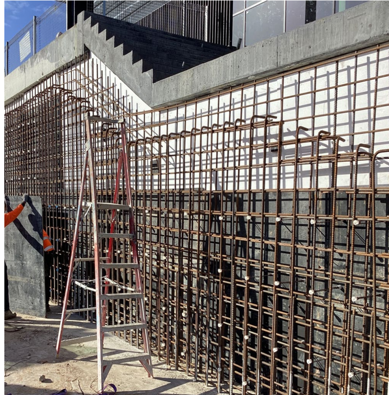
Northern Stair Steel & Formwork
