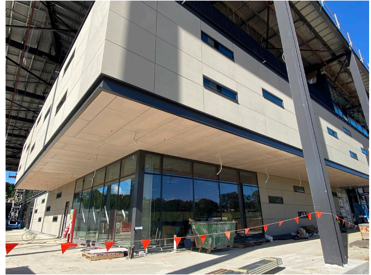
North-western corner – Soffit linings
