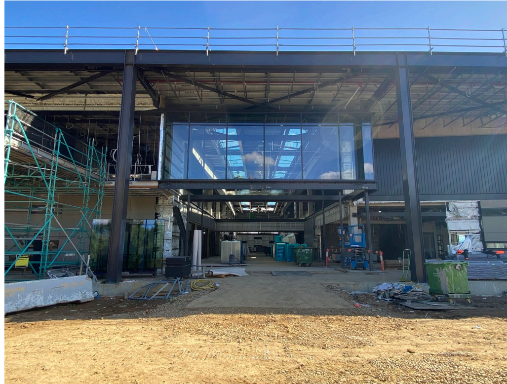
Eastern aspect – Glazing to Central Atrium Entry
