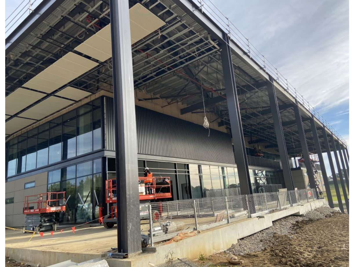
High-level soffit lining
