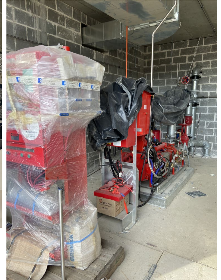
Fire system pump installation
