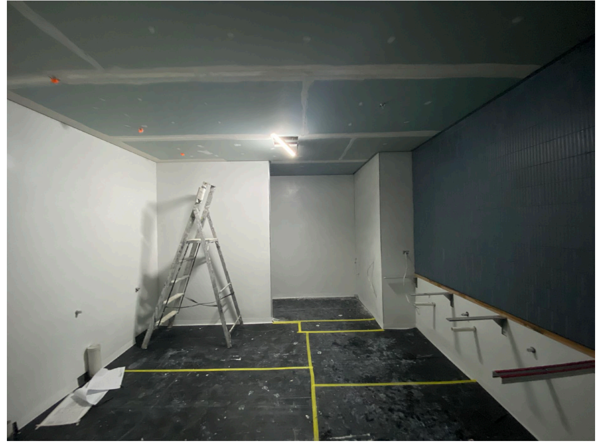
Amenity wall tiling completed and ceiling installed
