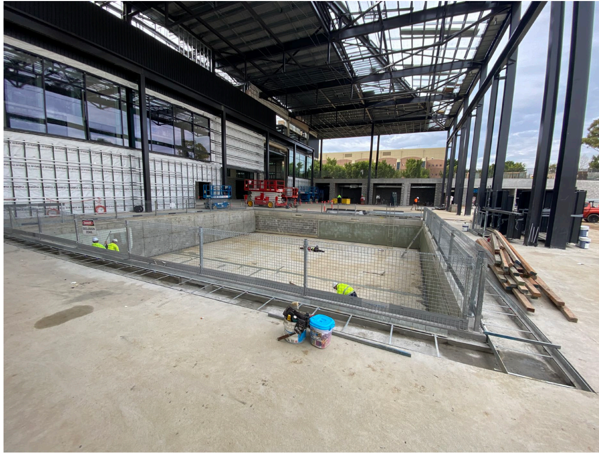
Waterproofing of Plumbing sandpit
