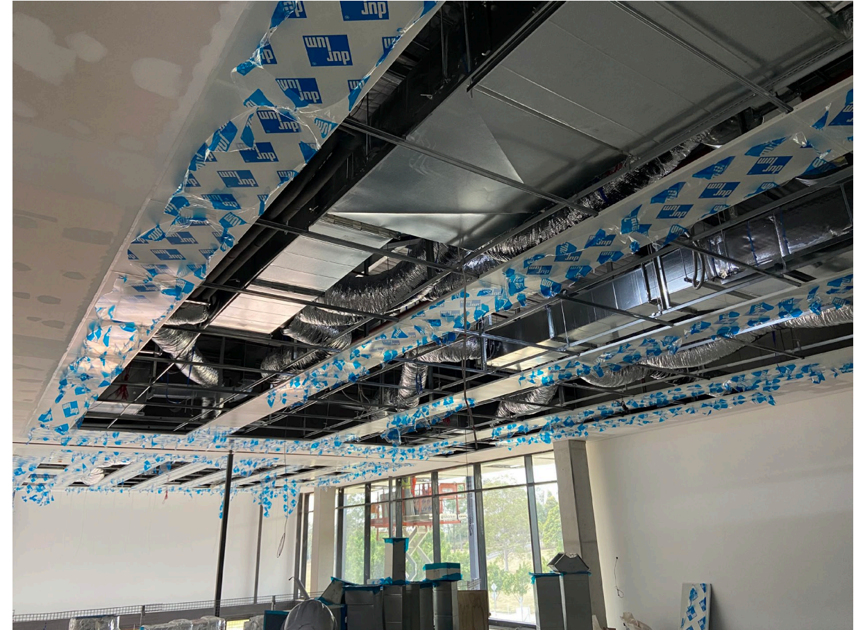
Closing up ceiling grids
