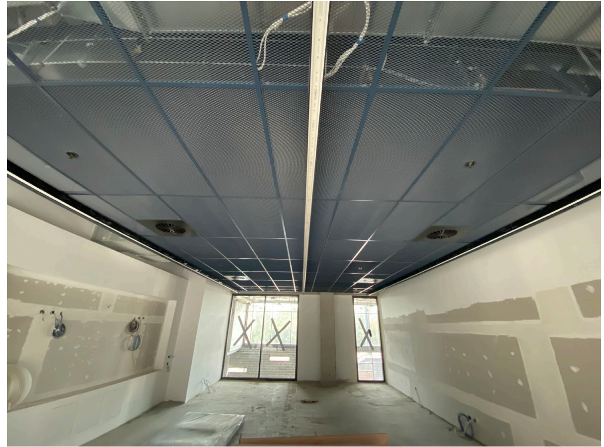
Ceiling grid and lighting installation
